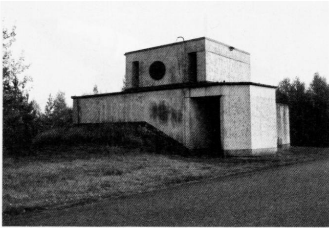
Well-protected building but of unknown use.
